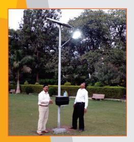
A standalone solar photovoltaic street lighting system comprises a compact fluorescent lamp lead acid battery, PV module/modules, control and control electronics, interconnecting wires /cables, Module mounting hardware, Battery box, and Operation instruction manual. We are offering Solar Street Lights.
